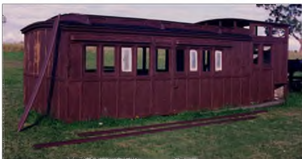
Work on the roof in progress while carriage on the ground
