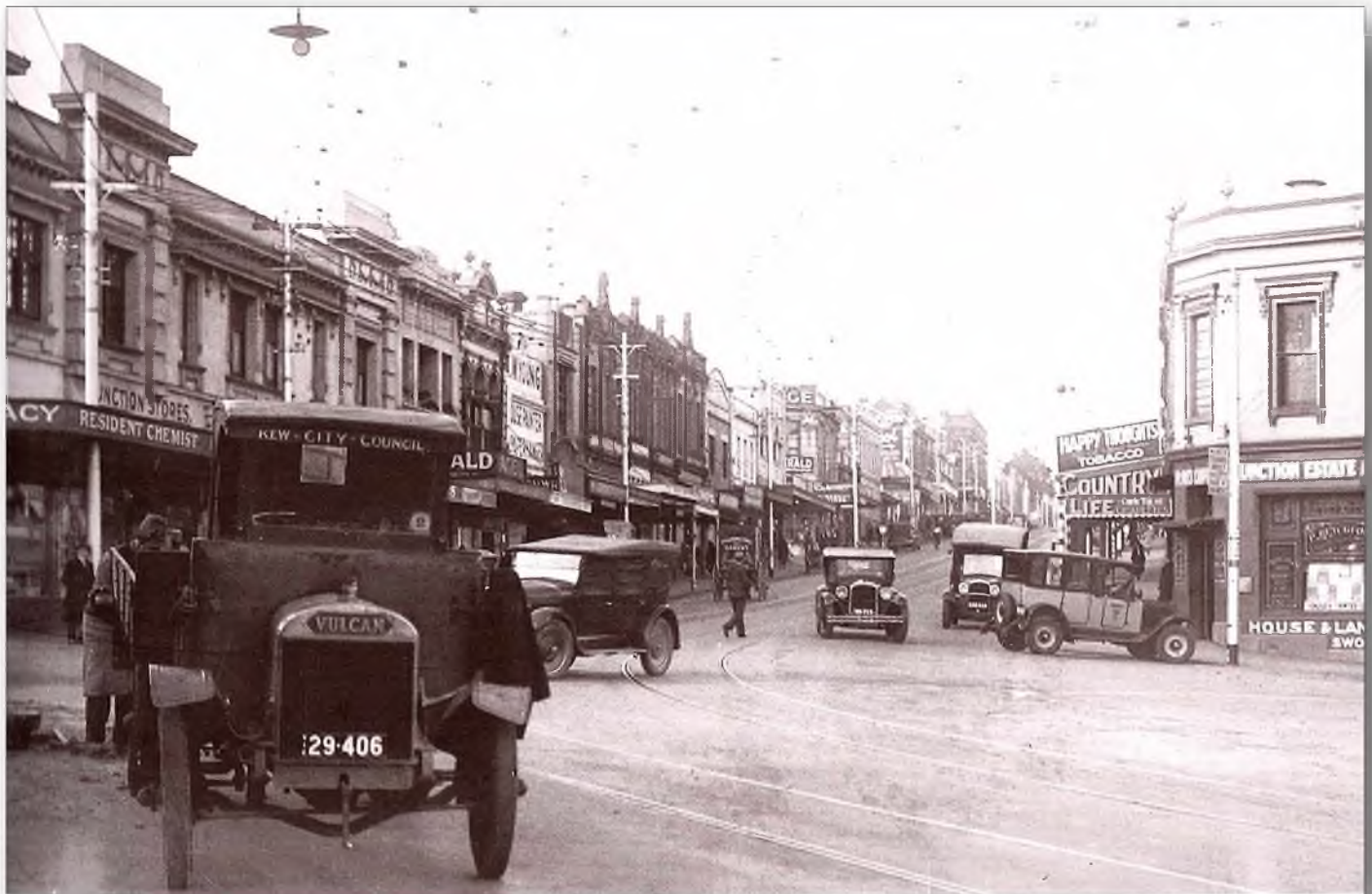
Kew Junction circa 1926-27 A Vulcan truck features prominently in this photograph evidently owned by the Kew City Council. It appears the council workers are repairing the road. No lights suggests it was only used during day light hours. In the back ground a Dodge Four tourer is trying to avoid the oddly parked Yellow cab. Taxi drivers have always been a law unto their own! Signage is interesting 'Happy Thoughts Tobacco'. Happy until you have lung cancer that is!
